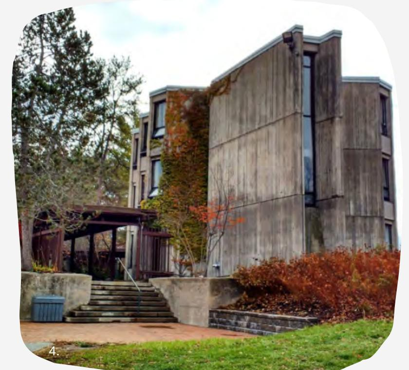
Lady Eaton College was constructed out of poured concrete and the walls were intentionally given a rough, board-marked finish. Originally, the College was to be built using the same rubble aggregate process as Champlain College, but this method proved too expensive. In total, Lady Eaton College cost \$3,917,000 to build, with this sum including all interior furnishings as well as external materials and contractor fees.
