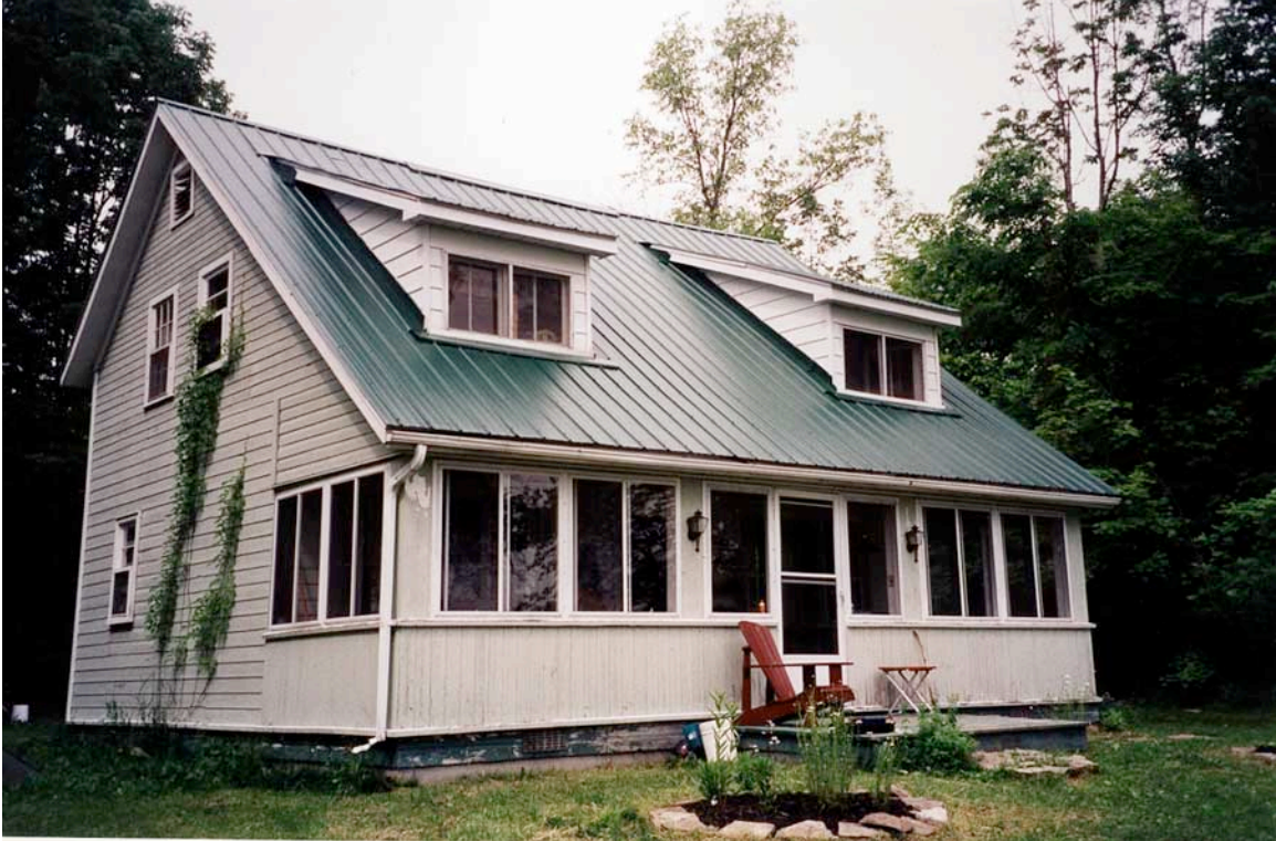
Plate 4. The Oliver Ecological Centre cottage was built in the early 1900's and now provides summer residence for researchers and field course participants. This cottage can accommodate up to fourteen researchers at one time. Photo Courtesy of Lois Davidson, June 2002.
